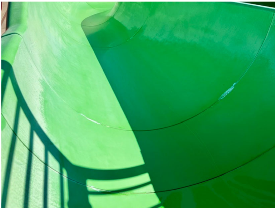
Spiral Slides finish and caulk
