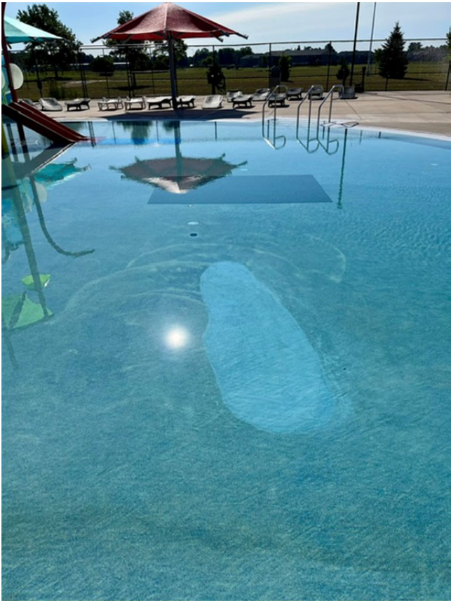
Recent plaster patches
